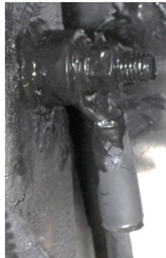
FIGURE 124: GROUND STUD WITH RUBBER COATING
