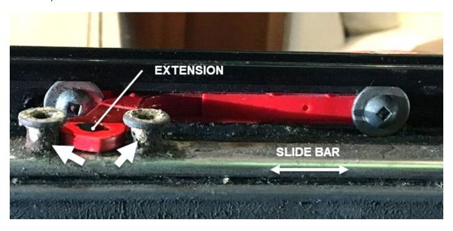
2. Remove the two (2) screws and remove the existing handle (see picture below).
