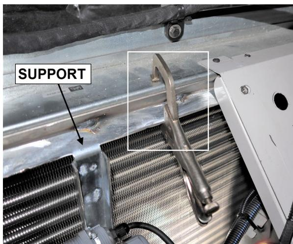
8. From the inside (using an angled drill), drill the two mounting holes in the housing (use the holes in the support tabs as a guide). Use a short 1/4 or 7/32 in (6mm) drill bit.
