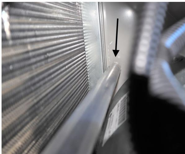
12. Using a sharpie, insert your hand and mark the tube position (perimeter of the tube).
