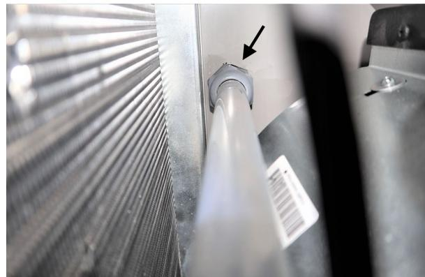
21. Hand tighten the four inner tube nuts to finalize the tubes installation in the evaporator housing.
