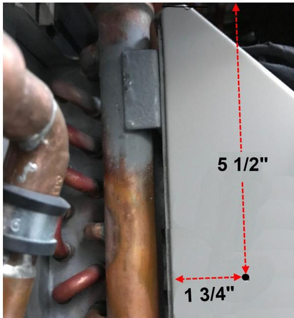
– Top tube pilot hole should be located approximately **5.5 in from the top** of the housing and the lower pilot hole **8.75 in from the top** (vertical positions).
