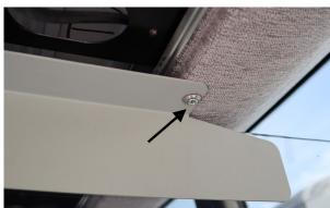
Using the partition top holes as a template, carefully drill corresponding holes in the top support (do not enlarge the partition holes with the drill).
