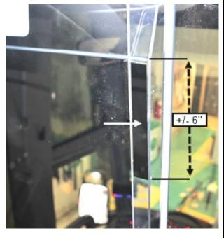
Drill a 6mm hole through both panels (and the foam tape) at the top corner where the two panels are making contact (+/- 3in from the top of the foam tape strip).
