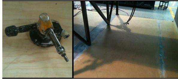
15. Apply adhesive 8714628 over plywood surface.
