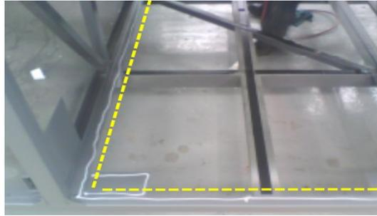
11. Reuse the old plywood as shape reference in order to mark the perimeter of the cutouts on the new plywood.
