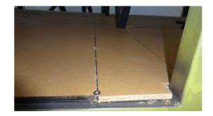
13. Mix the sealant and catalyst 8715036, and then apply it on the wood imperfections in order to have a flat surface.
