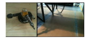
15. Apply adhesive 8714628 over plywood surface.
