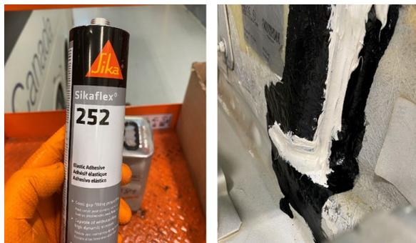
6. 6. Apply the second layer of Primer-206 and Sikaflex-252 over the area of the leak.
