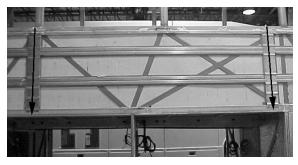
Install a neoprene foam tape at the center of panel horizontal supports and at each end if needed.
