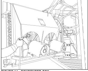
FIGURE 14: CONDENSER COIL
