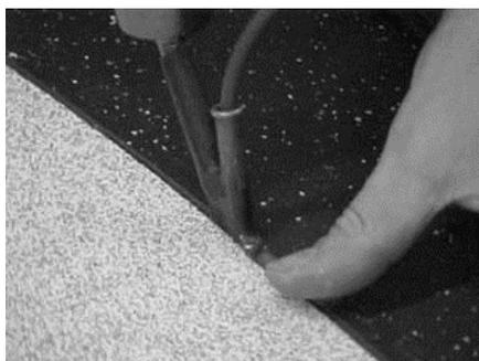
4. Always add an extra inch of filler bead at the beginning and at the end of repair.
