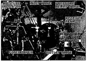
Figure 24: A/C Condenser Compartment
