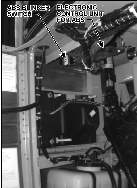
FIGURE 34: STEERING COMPARTMENT (LEFT WALL) 06119
