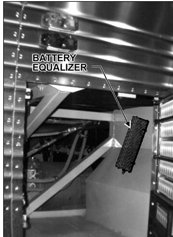
FIGURE 45: R.H. SIDE REAR SERVICE COMPARTMENT
