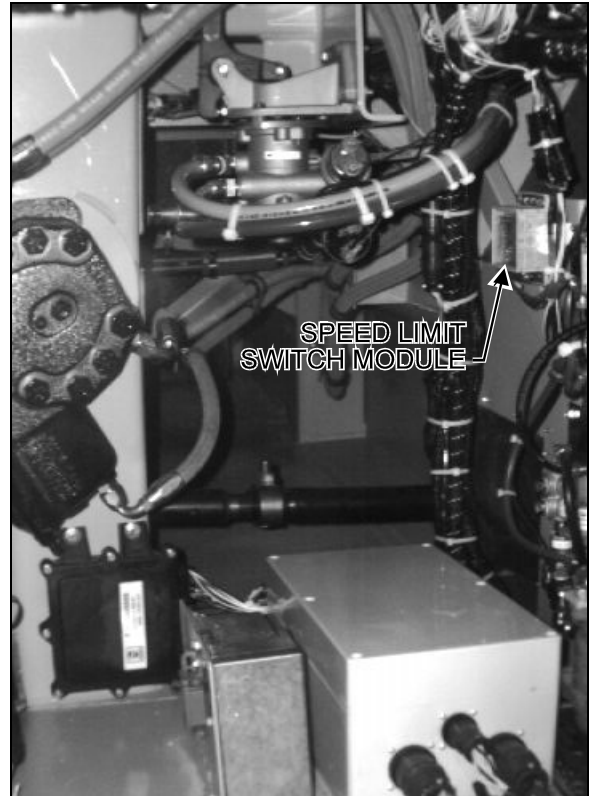
FIGURE 36: STEERING COMPARTMENT (RIGHT WALL) 06169
