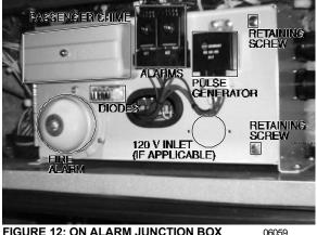
FIGURE 12: ON ALARM JUNCTION BOX
