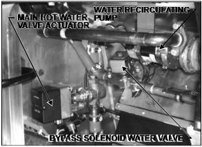
FIGURE 34: HVAC COMPARTMENT
