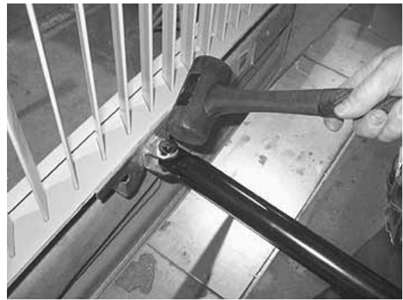
FIGURE 61: DOOR LATERAL ADJUSTMENT
