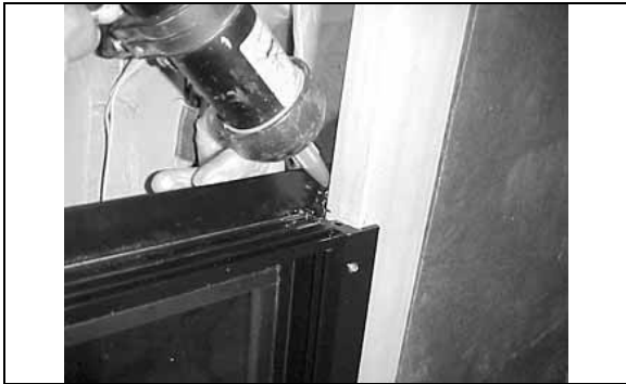
FIGURE 79 : SLIDING WINDOW – SEAL THE UPPER CORNERS
