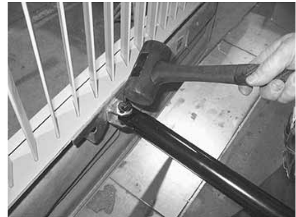
FIGURE 65: DOOR LATERAL ADJUSTMENT
