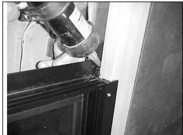
FIGURE 73 : AWNING WINDOW – SEAL THE UPPER CORNERS
