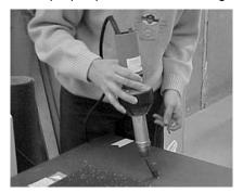
7. Once the welding torch is ready, insert the filler bead into the nozzle and immediately start welding. Move in a regular manner while pressing slightly with torch.
