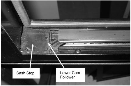
FIGURE 24: PROPER ALIGNMENT
