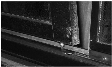
FIGURE 23: DISENGAGING THE BOTTOM OF THE SASH
