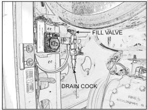
FIGURE 2: REAR VALVE LOCATION (TYPICAL)
