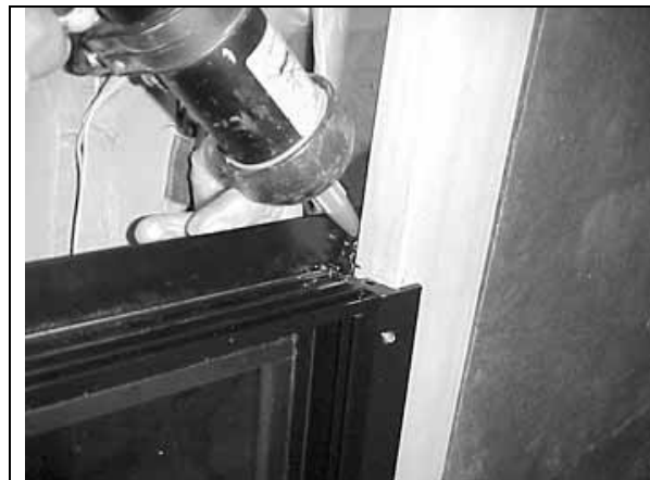
FIGURE 73 : AWNING WINDOW – SEAL THE UPPER CORNERS
