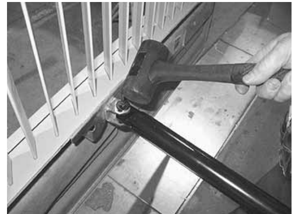
FIGURE 71: DOOR LATERAL ADJUSTMENT
