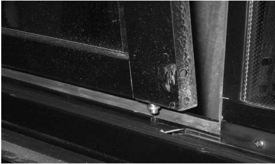
FIGURE 42: DISENGAGING THE BOTTOM OF THE SASH
