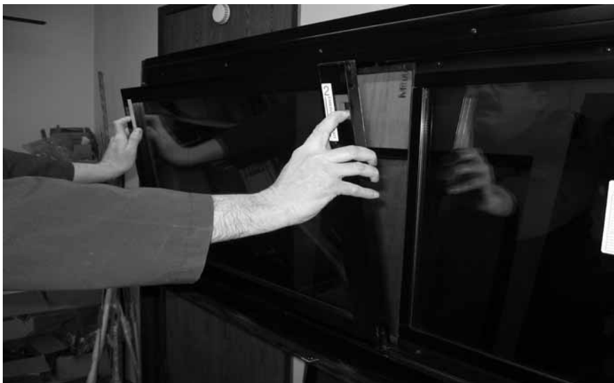
FIGURE 41: REMOVING THE SASH
