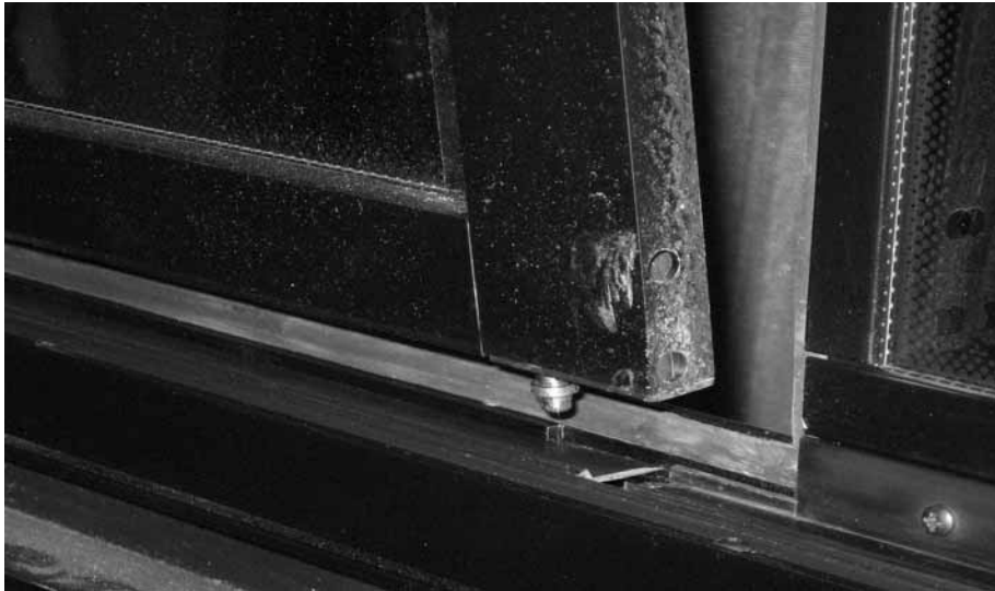
FIGURE 42: DISENGAGING THE BOTTOM OF THE SASH
