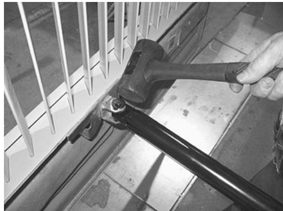
FIGURE 64: DOOR LATERAL ADJUSTMENT
