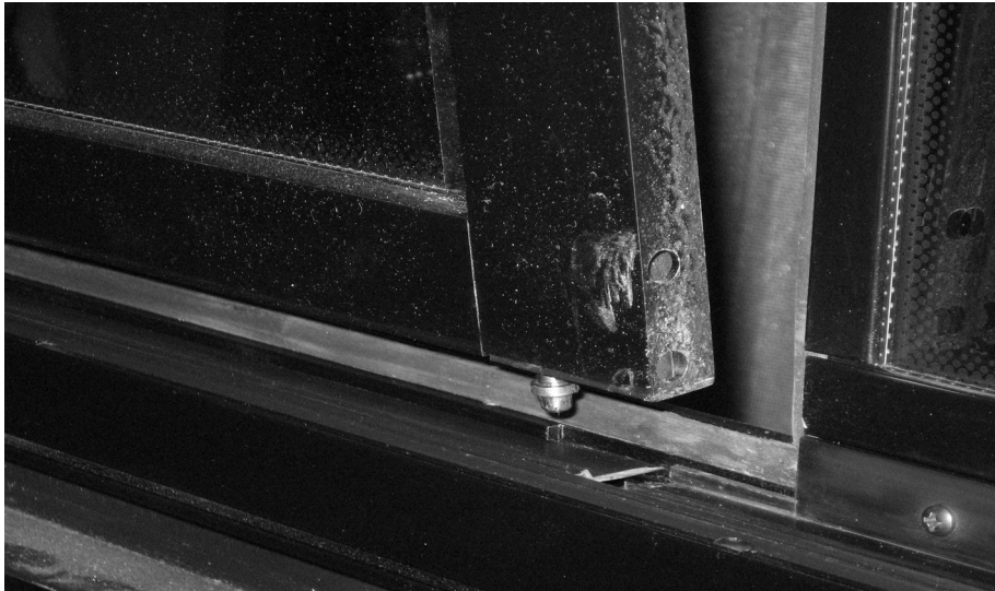
FIGURE 42: DISENGAGING THE BOTTOM OF THE SASH
