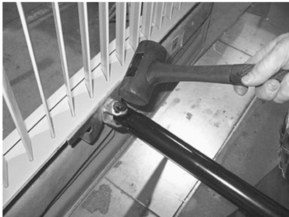
FIGURE 64: DOOR LATERAL ADJUSTMENT
