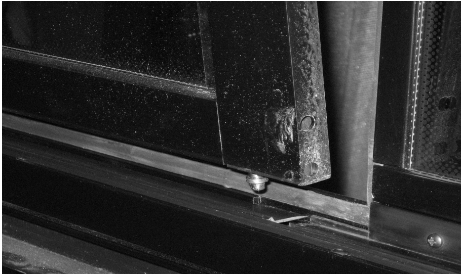
FIGURE 42: DISENGAGING THE BOTTOM OF THE SASH
