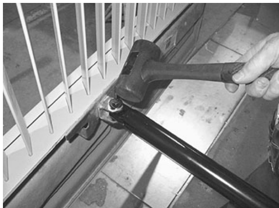
FIGURE 65: DOOR LATERAL ADJUSTMENT
