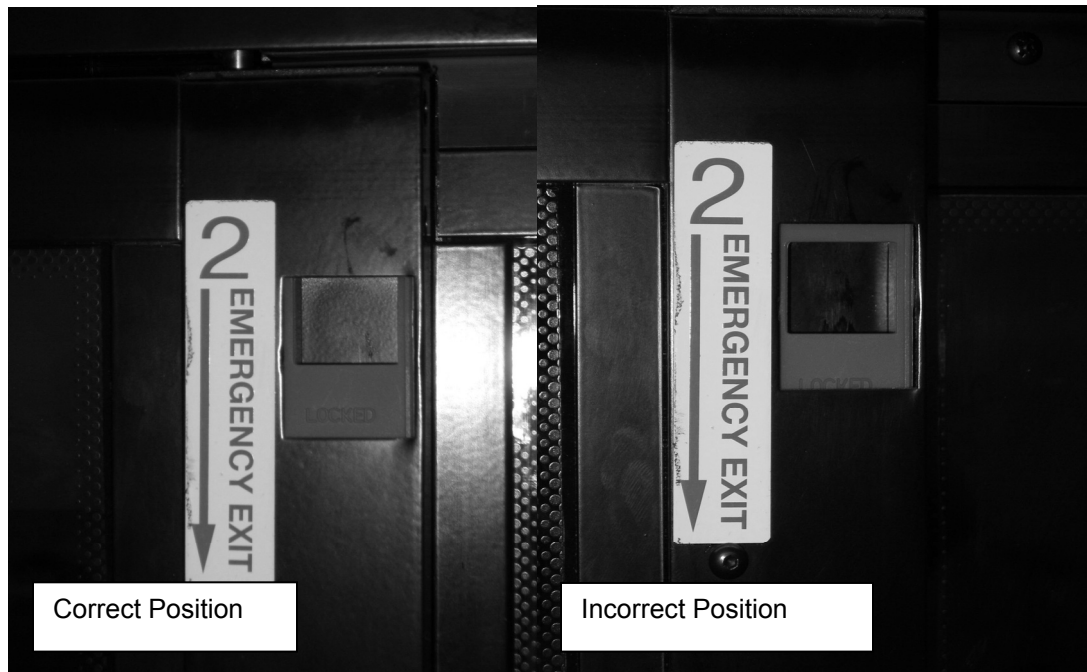
FIGURE 25: RELEASE LATCH PROPER POSITION
