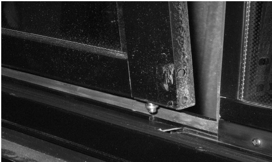
FIGURE 22: DISENGAGING THE BOTTOM OF THE SASH
