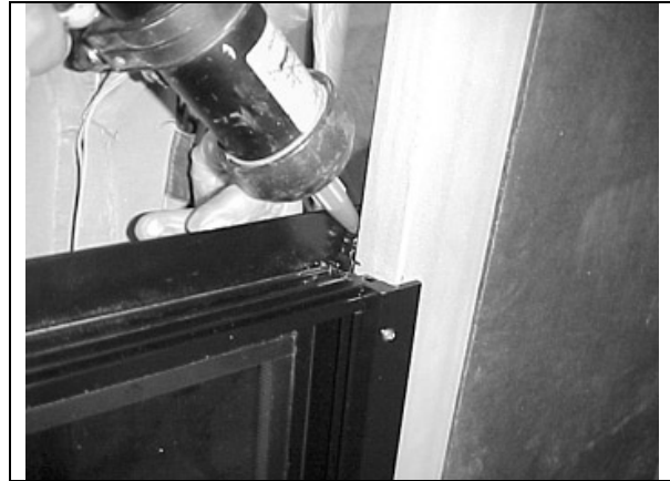
FIGURE 75 : SLIDING WINDOW – SEAL THE UPPER CORNERS
