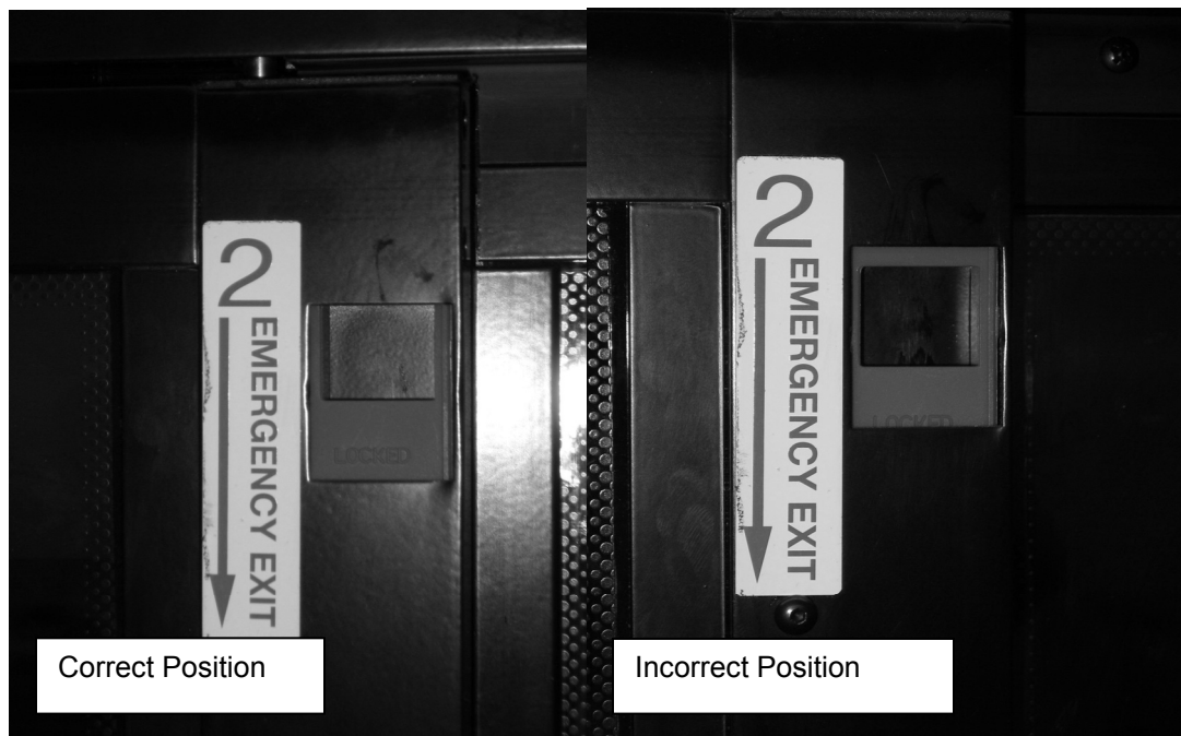
FIGURE 25: RELEASE LATCH PROPER POSITION
