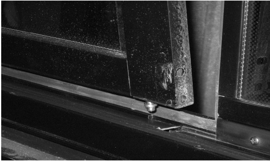
FIGURE 42: DISENGAGING THE BOTTOM OF THE SASH
