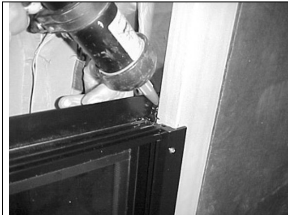
FIGURE 74 : AWNING WINDOW – SEAL THE UPPER CORNERS
