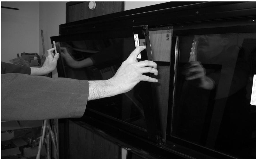
FIGURE 41: REMOVING THE SASH
