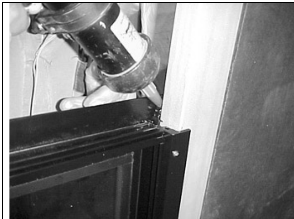
FIGURE 69 : AWNING WINDOW – SEAL THE UPPER CORNERS
