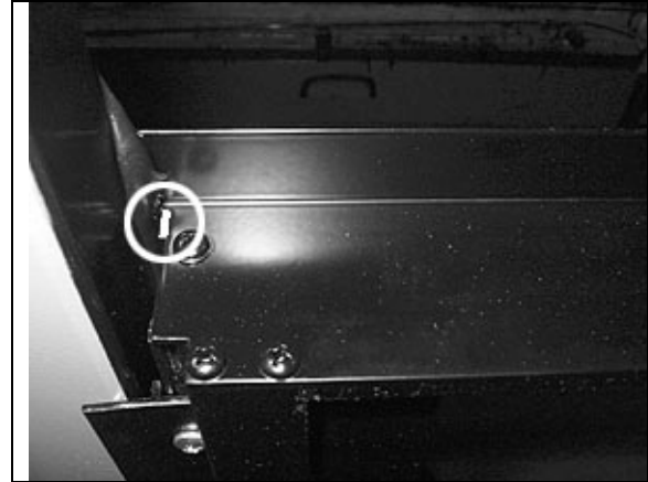
FIGURE 70 : AWNING WINDOW – SEAL THE CHINK
