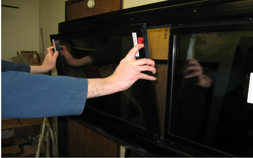
FIGURE 62: REMOVING THE SASH
