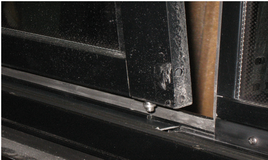
FIGURE 63: DISENGAGING THE BOTTOM OF THE SASH
