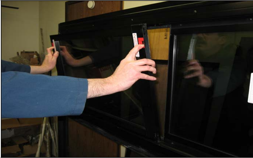
FIGURE 64: REMOVING THE SASH
