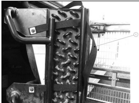
CONDENSER COMPARTMENT STRAP
