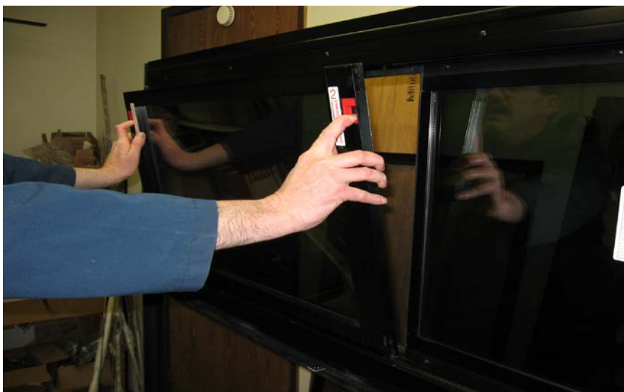
FIGURE 50: REMOVING THE SASH
