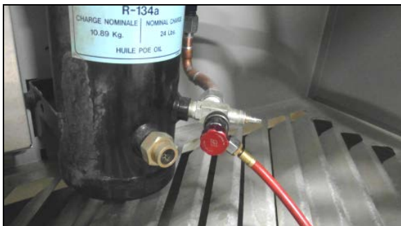
FIGURE 78: RECOVERY UNIT CONNECTED TO RECEIVER SERVICE PORT
