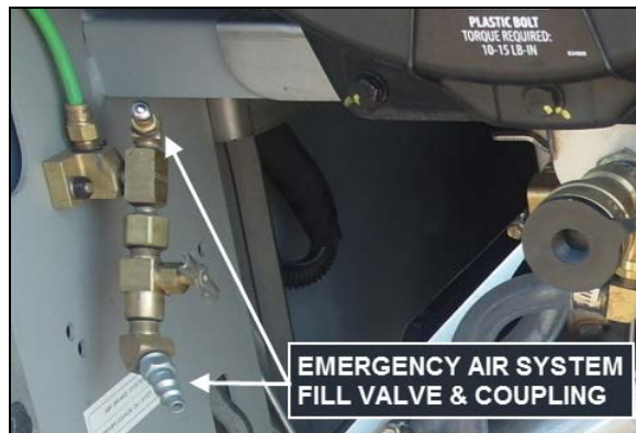
EMERGENCY AIR SYSTEM FILL VALVE AND COUPLING
