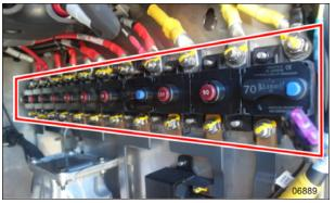
MAIN CIRCUIT BREAKERS IN MPC
