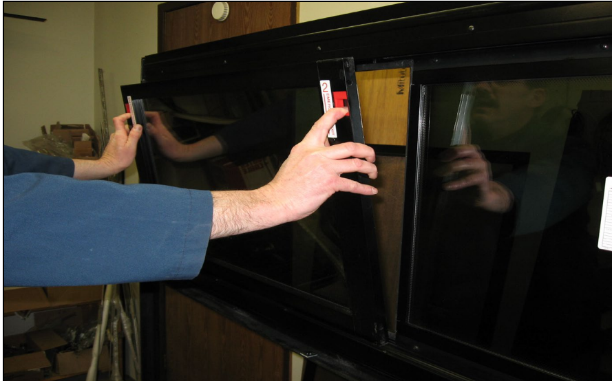
FIGURE 107: REMOVING THE SASH
