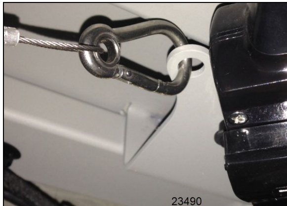
FIGURE 46: PROTECTIVE WIRE INSTALLATION
