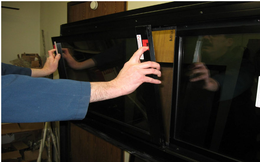
FIGURE 47: REMOVING THE SASH
