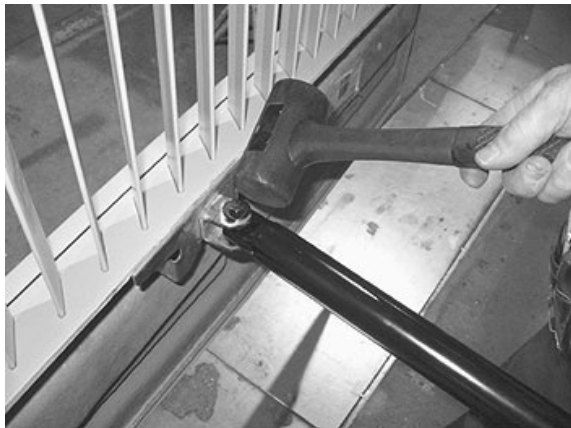
FIGURE 85: DOOR LATERAL ADJUSTMENT
