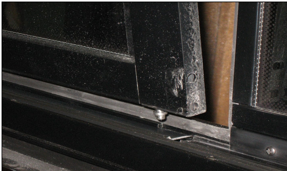
FIGURE 108: DISENGAGING THE BOTTOM OF THE SASH
