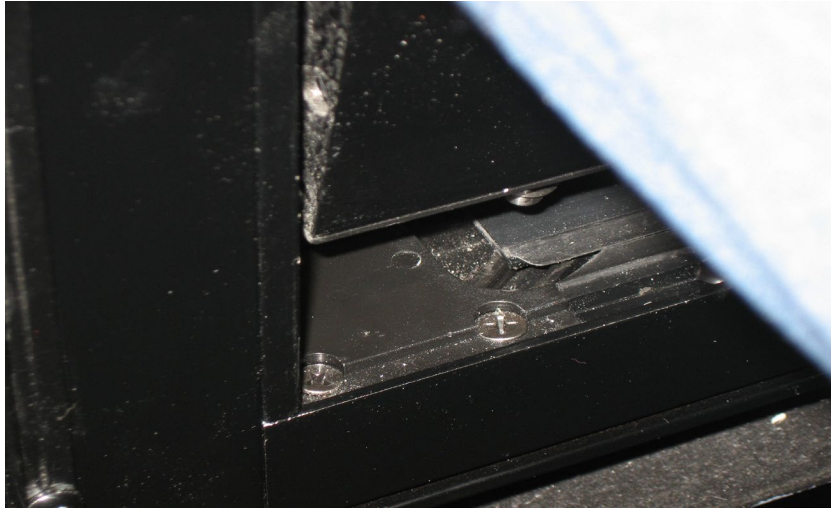
FIGURE 50: POSITIONING THE LOWER LEFT CORNER OF THE SASH
