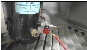
FIGURE 98: RECOVERY UNIT CONNECTED TO RECEIVER SERVICE PORT
