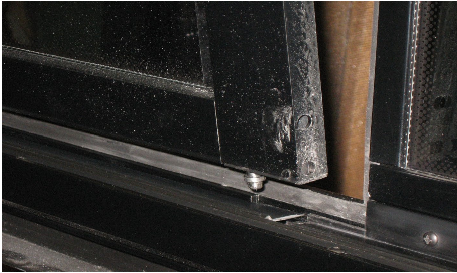
FIGURE 48: DISENGAGING THE BOTTOM OF THE SASH
