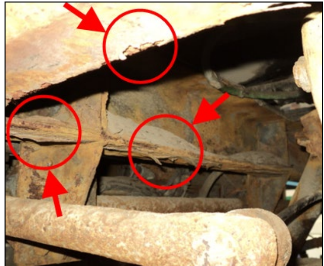
FIGURE 3: METAL FLAKING AND ACCUMULATED SAND
