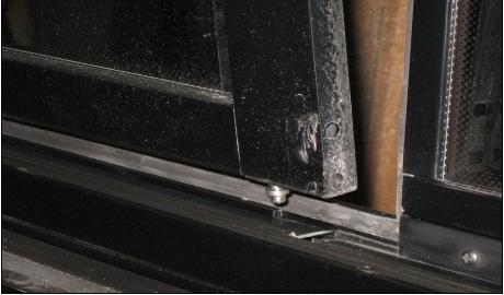
FIGURE 108: DISENGAGING THE BOTTOM OF THE SASH
