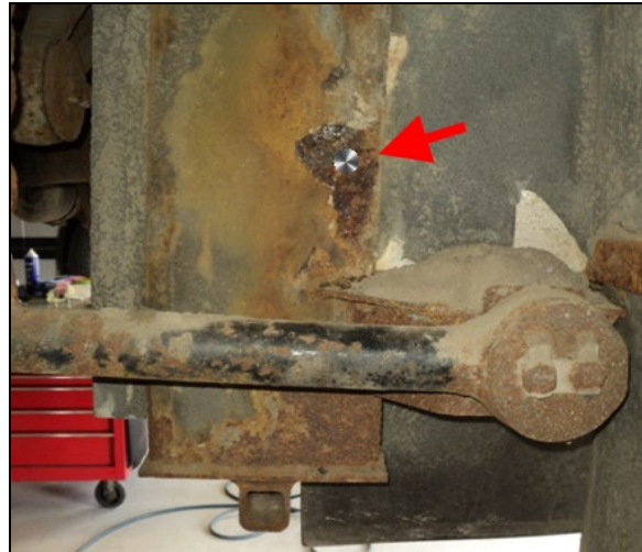
FIGURE 6: CLEANED SPOT ON STRUCTURAL MEMBER
