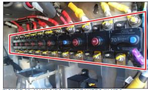
FIGURE 25: MAIN CIRCUIT BREAKERS IN MPC
