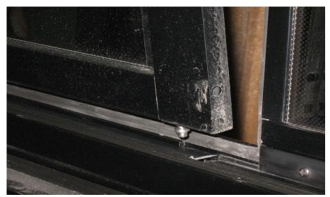
FIGURE 48: DISENGAGING THE BOTTOM OF THE SASH
