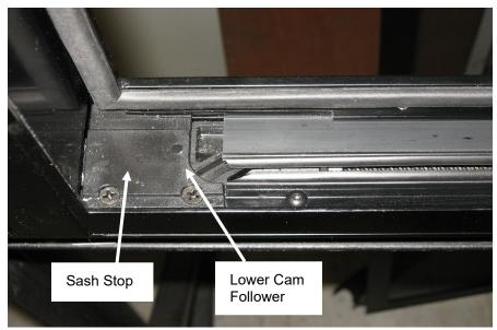
FIGURE 49: PROPER ALIGNMENT
