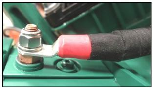
Figure 19: No exposed or broken copper strands.
