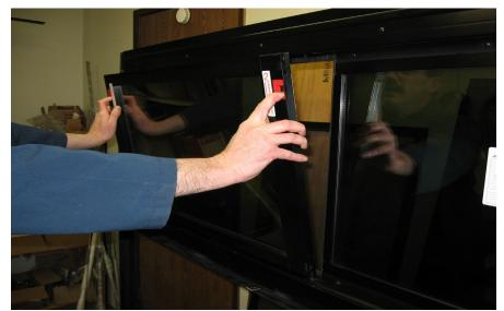
FIGURE 47: REMOVING THE SASH
