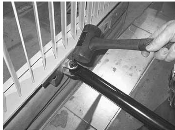
FIGURE 61: DOOR LATERAL ADJUSTMENT
