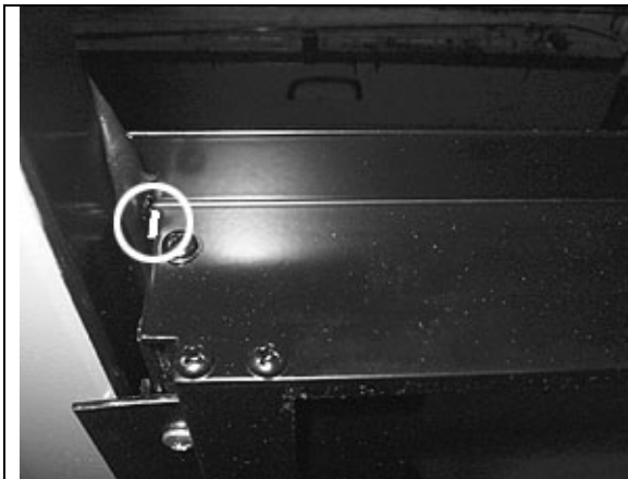
FIGURE 70 : AWNING WINDOW – SEAL THE CHINK
