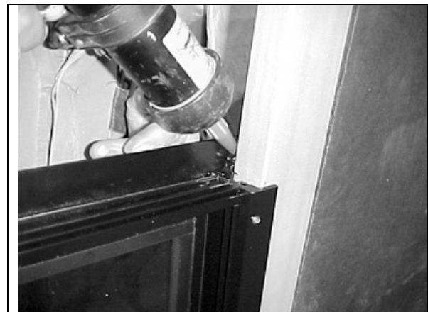
FIGURE 69 : AWNING WINDOW – SEAL THE UPPER CORNERS
