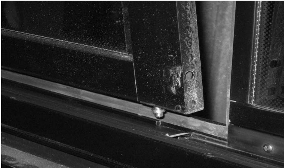
FIGURE 42: DISENGAGING THE BOTTOM OF THE SASH
