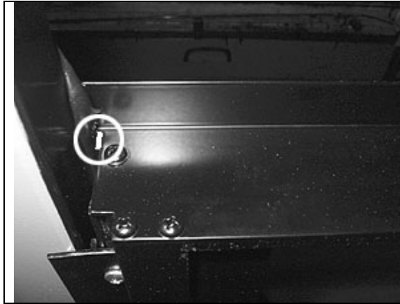
FIGURE 74 : AWNING WINDOW – SEAL THE CHINK
