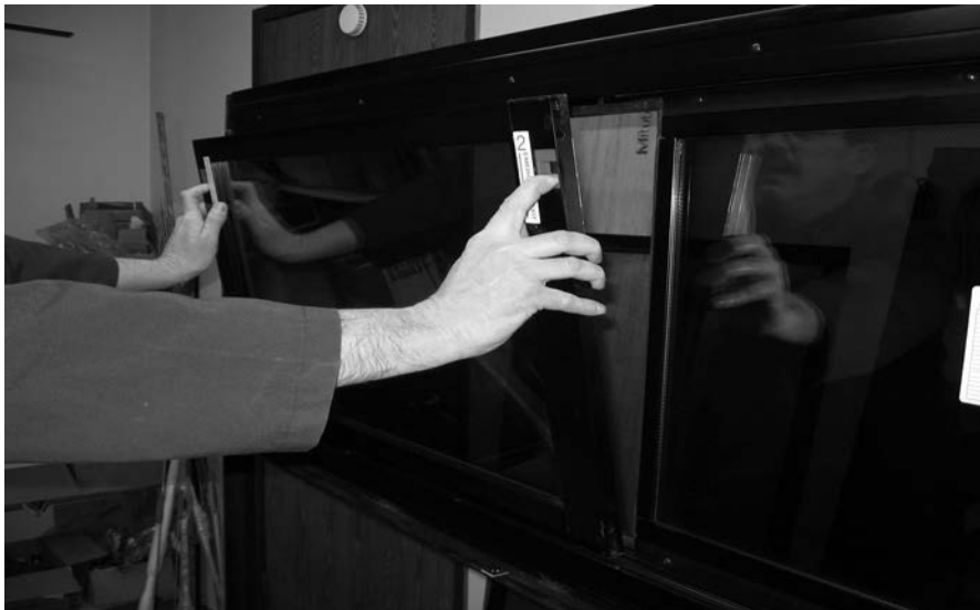
FIGURE 41: REMOVING THE SASH
