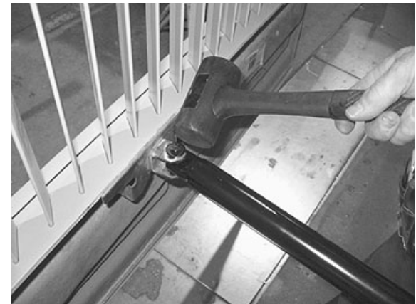
FIGURE 71: DOOR LATERAL ADJUSTMENT
