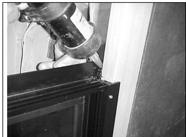
FIGURE 73 : AWNING WINDOW – SEAL THE UPPER CORNERS
