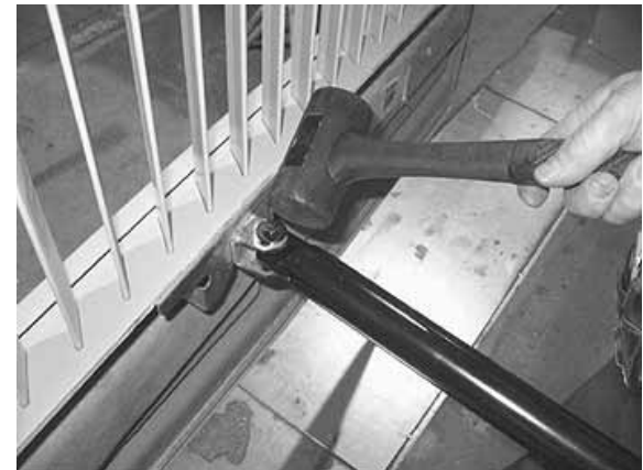
FIGURE 71: DOOR LATERAL ADJUSTMENT
