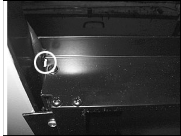
FIGURE 75 : AWNING WINDOW – SEAL THE CHINK
