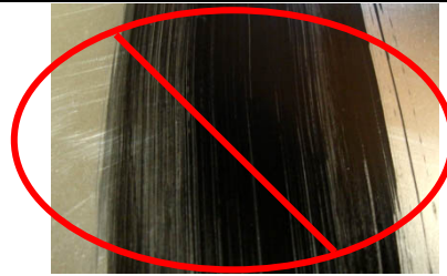
Uneven. Apply again locally onto missing areas after waiting drying time
