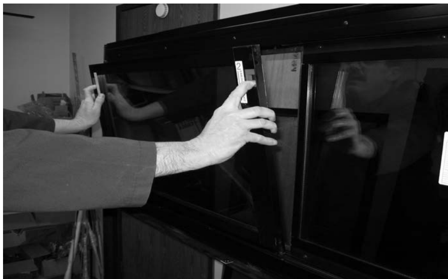
FIGURE 21: REMOVING THE SASH
