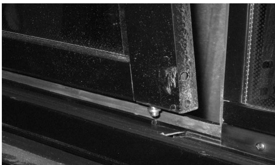
FIGURE 22: DISENGAGING THE BOTTOM OF THE SASH
