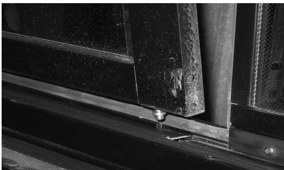
FIGURE 22: DISENGAGING THE BOTTOM OF THE SASH
