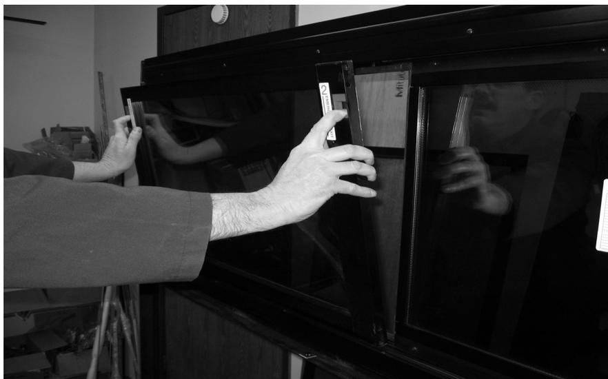
FIGURE 21: REMOVING THE SASH
