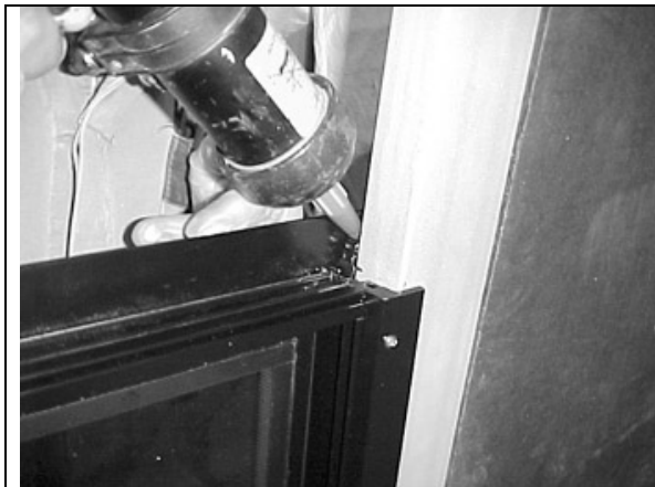
FIGURE 69 : AWNING WINDOW – SEAL THE UPPER CORNERS
