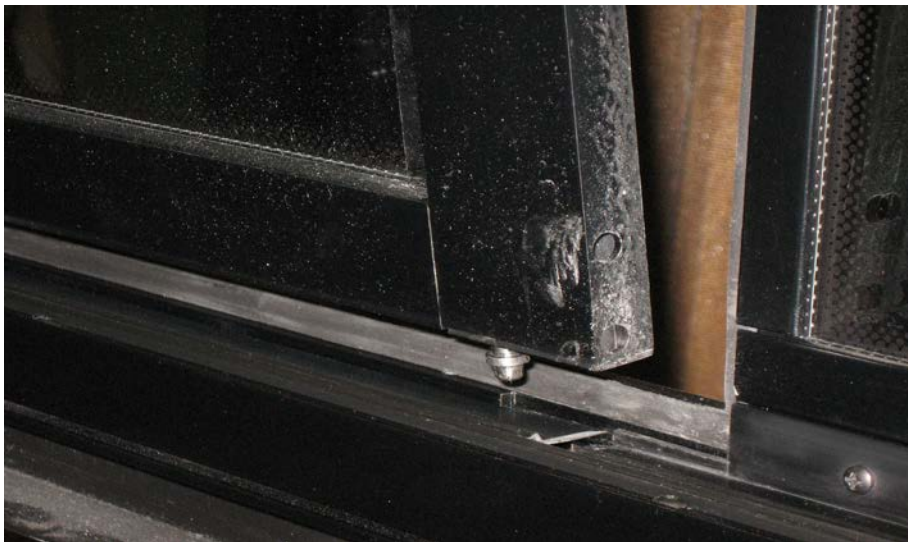
FIGURE 63: DISENGAGING THE BOTTOM OF THE SASH
