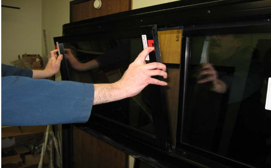
FIGURE 62: REMOVING THE SASH
