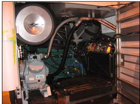
FIGURE 7: REAR ELECTRICAL PANEL, JUNCTION PANEL & BATTERY COMPARTMENT
