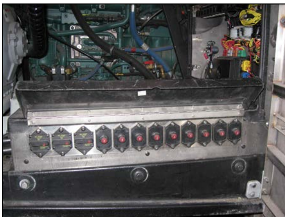
FIGURE 10: REAR ELECTRICAL JUNCTION PANEL 06634
