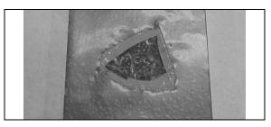
Using a plastic spatula, apply some Sika 221 grey onto the damaged area.
