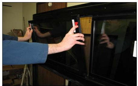
FIGURE 64: REMOVING THE SASH
