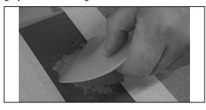
Remove masking tape and protection around damaged area.
