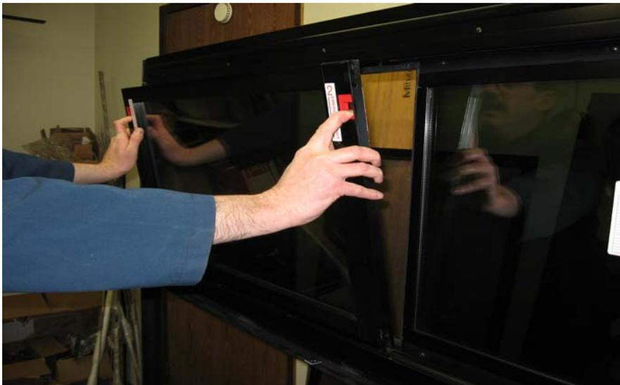
FIGURE 41: REMOVING THE SASH
