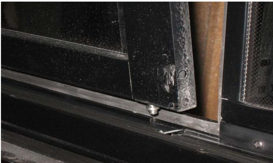
FIGURE 42: DISENGAGING THE BOTTOM OF THE SASH
