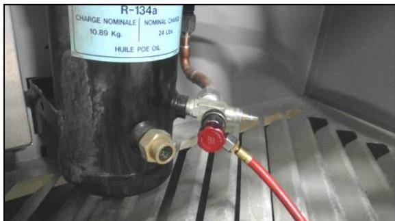
FIGURE 80: RECOVERY UNIT CONNECTED TO RECEIVER SERVICE PORT
