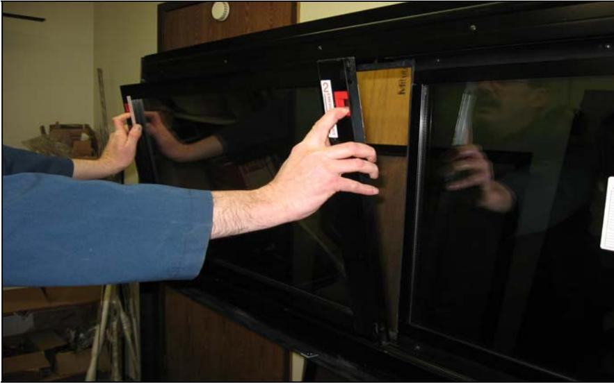
**FIGURE 64: REMOVING THE SASH**
