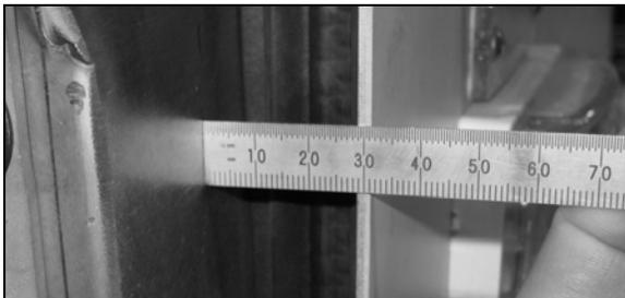
5. Respect the required gap between exterior finishing panels.
