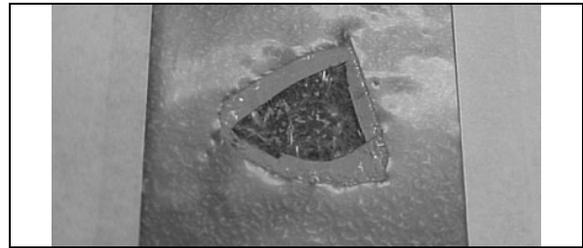
Using a plastic spatula, apply some Sika 221 grey onto the damaged area.
