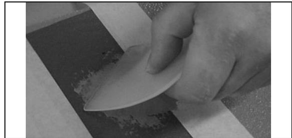
Remove masking tape and protection around damaged area.
