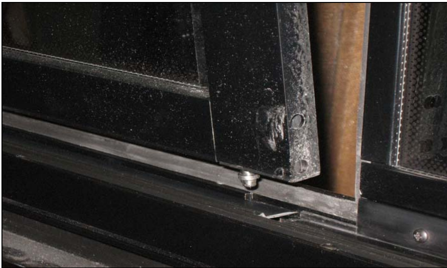
FIGURE 65: DISENGAGING THE BOTTOM OF THE SASH
