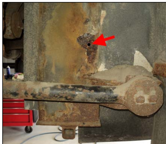
FIGURE 7: HOLE DRILLED IN STRUCTURAL MEMBER
