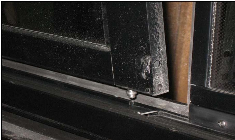
FIGURE 96: DÉGAGEMENT DU BAS DU CHÂSSIS
