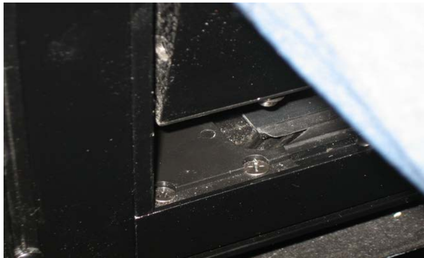
FIGURE 53: POSITIONING THE LOWER LEFT CORNER OF THE SASH
