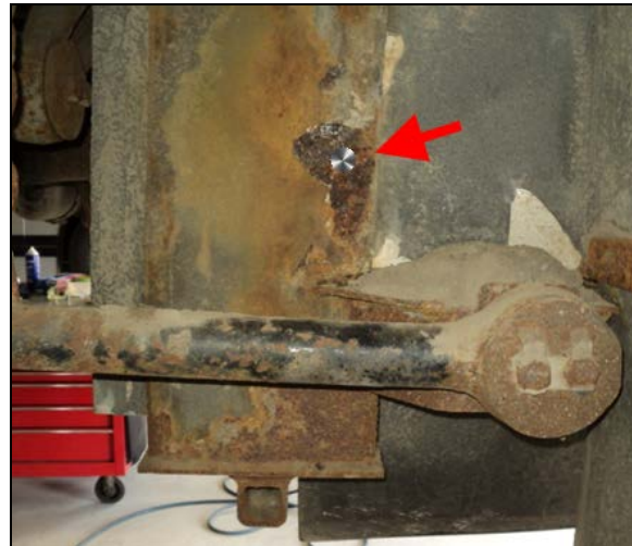
FIGURE 6: CLEANED SPOT ON STRUCTURAL MEMBER
