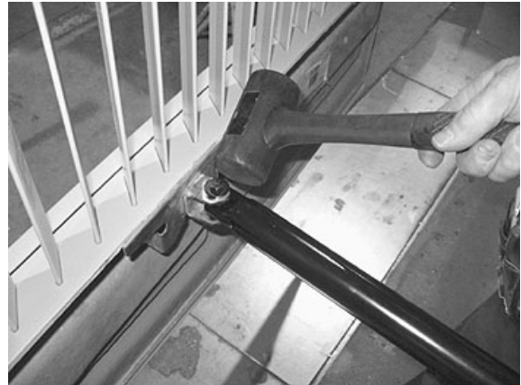
FIGURE 73: DOOR LATERAL ADJUSTMENT
