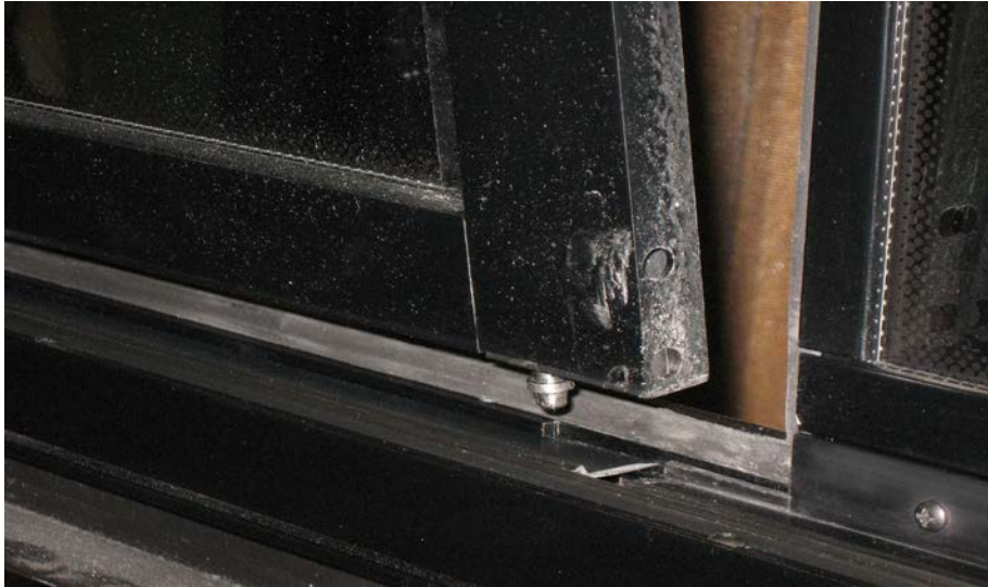
FIGURE 51: DISENGAGING THE BOTTOM OF THE SASH
