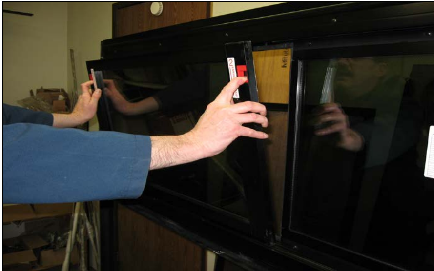
FIGURE 95: REMOVING THE SASH
