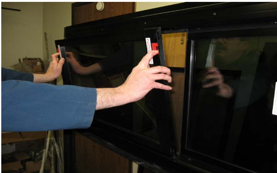
FIGURE 50: REMOVING THE SASH
