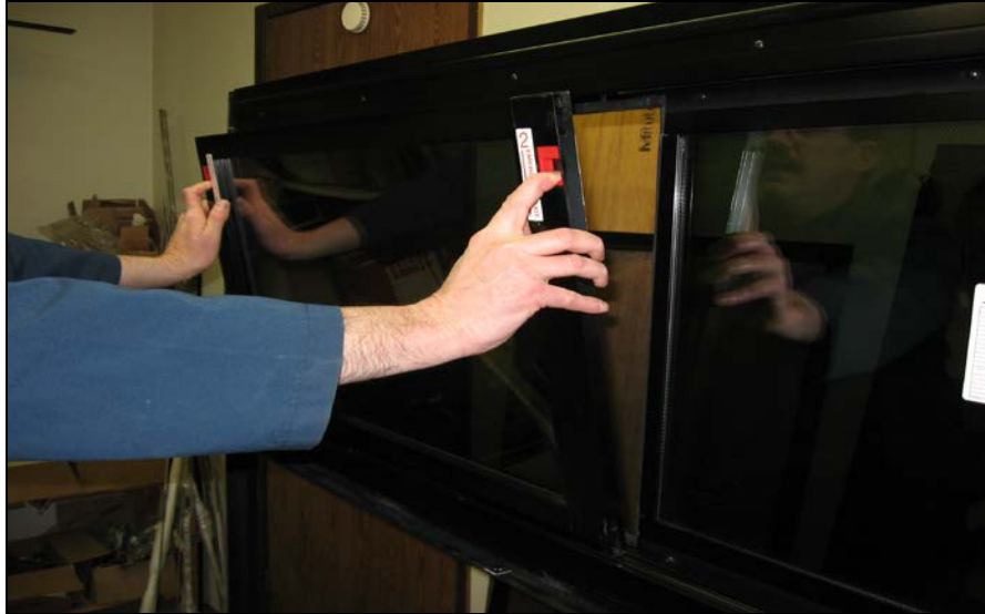
FIGURE 95: REMOVING THE SASH
