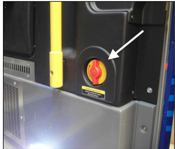
INTERIOR EMERGENCY RELEASE AIR VALVE
