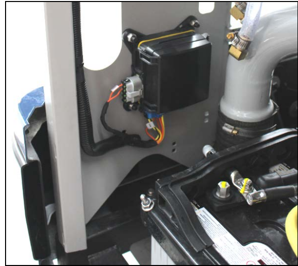
FIGURE 45: VECT (CURB SIDE)
